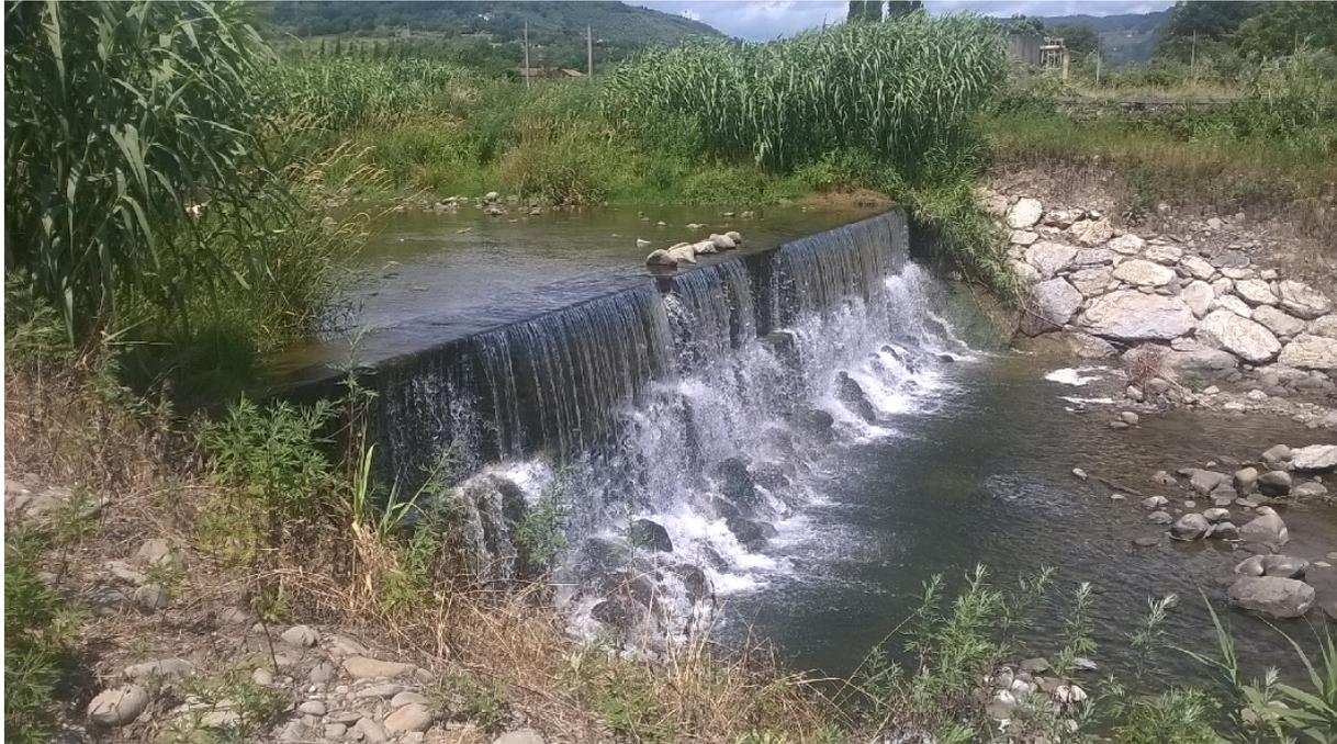
FIGURA 2. SALTO DI FONDO SUL T. PESCIA DI COLLODI (INLINE STRUCTURE N. 51.5)
